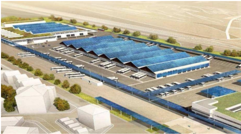
Figure 5-1- Dijon's bus/tram depot comprises a 1.5 MW solar panel roof installation (2012)
